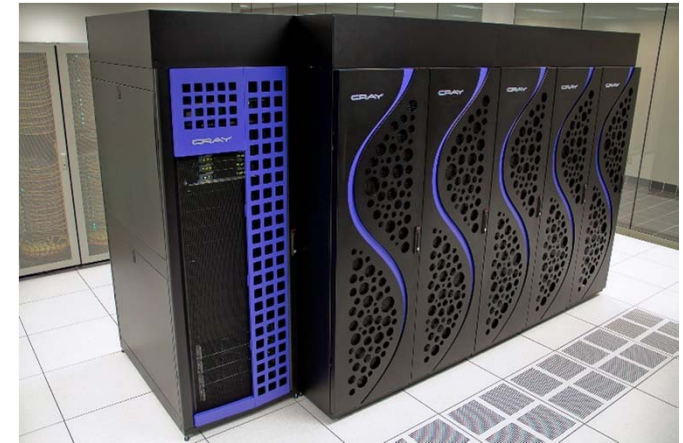
Cray installation at Mississippi State University with Asetek RackCDU
